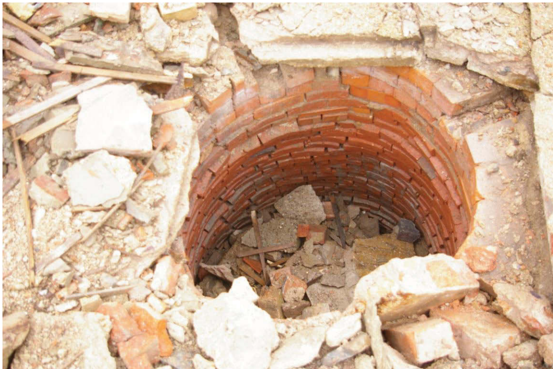
Figure 3: Cold water tank
