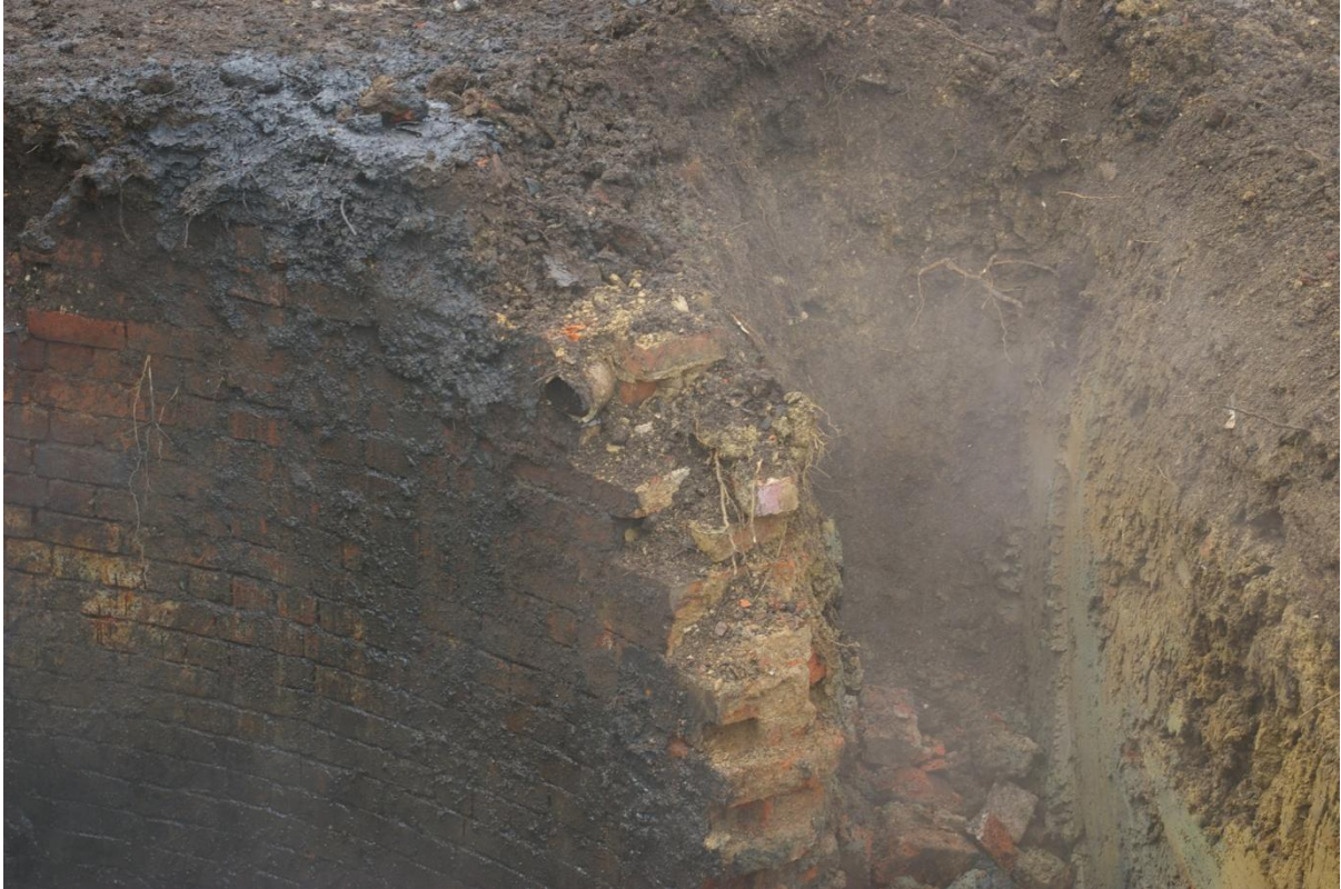
Figure 7: Detailed view of brick structure
