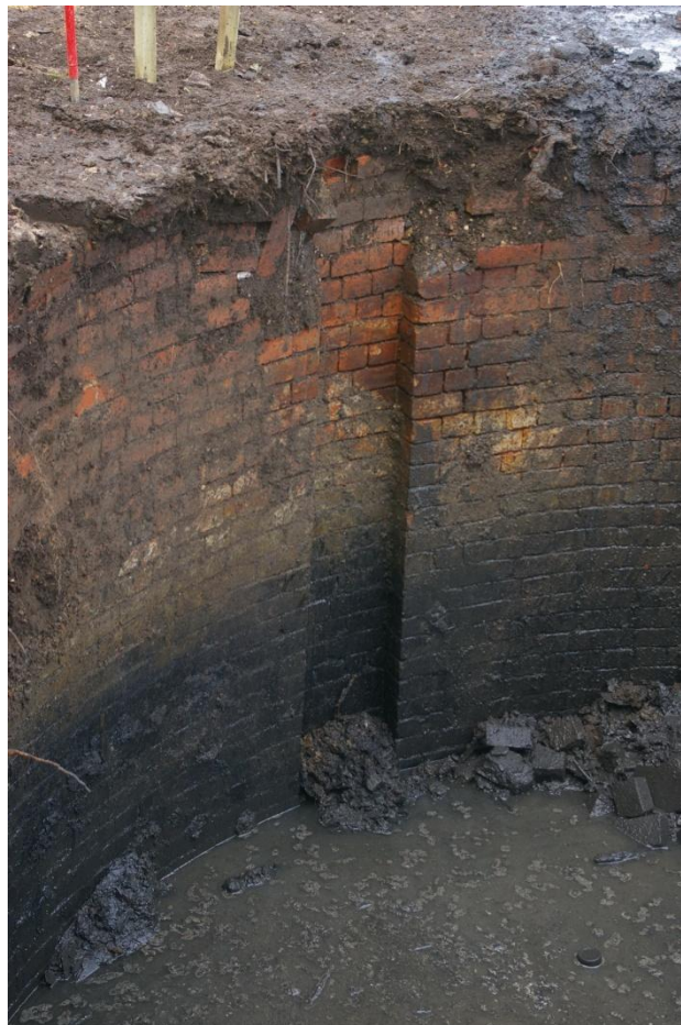
Figure 6: Detailed view of brick structure
