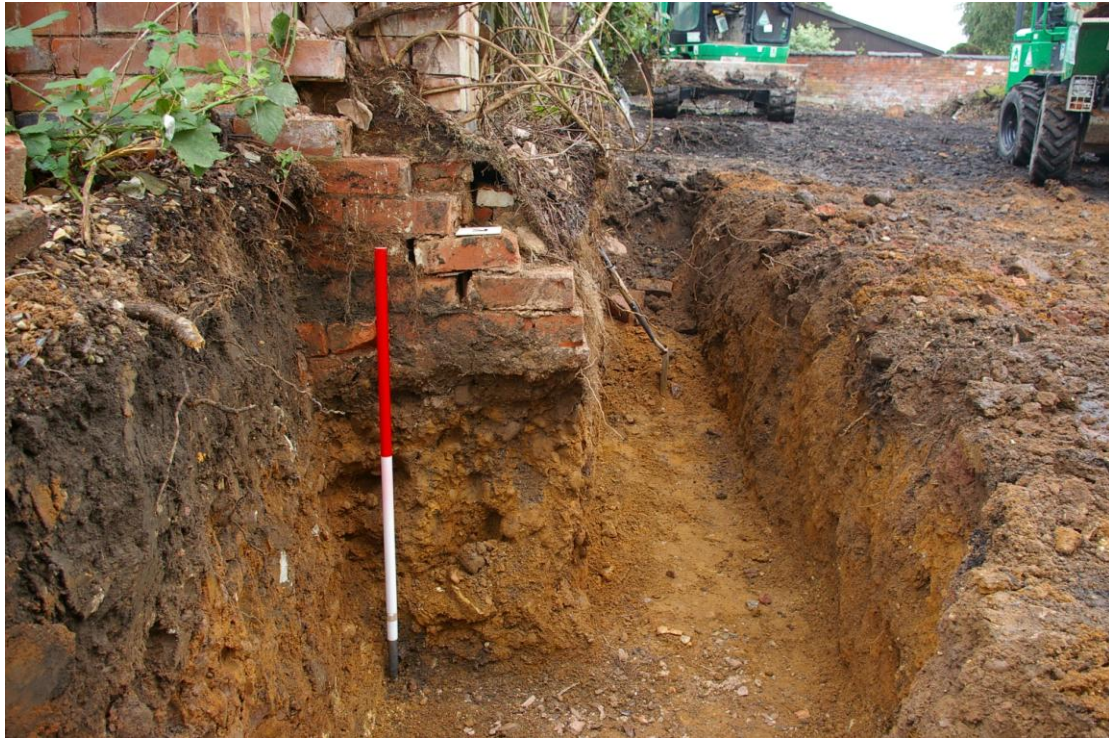
Plate 3: Trenches against neighbouring property, looking south-west
