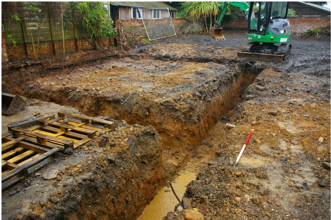
Plate 6: Foundations completed, looking south
