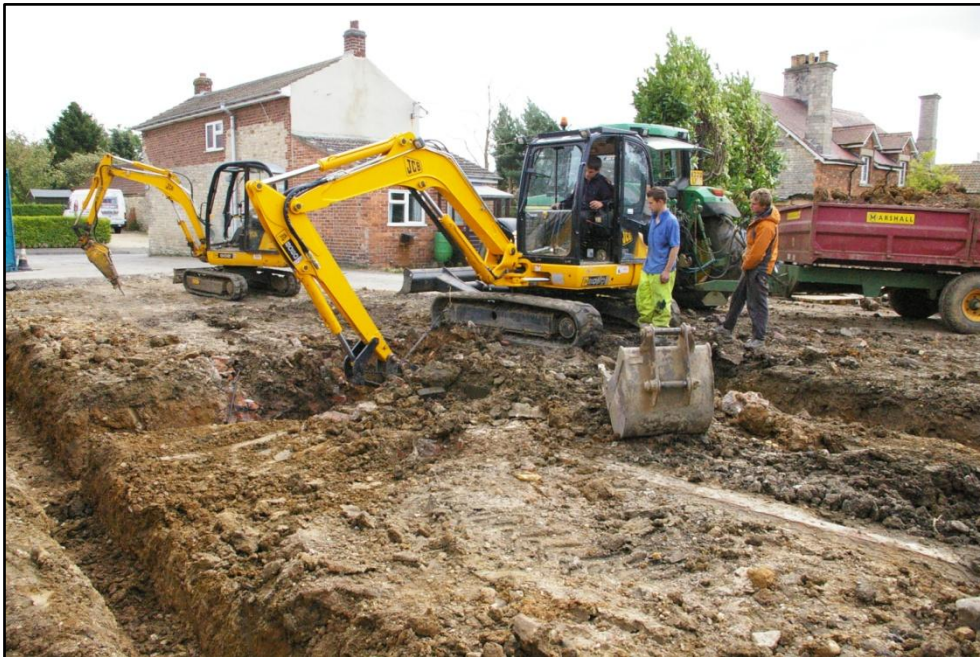
Plate 2: Machine excavating foundation trenches for plot 3
