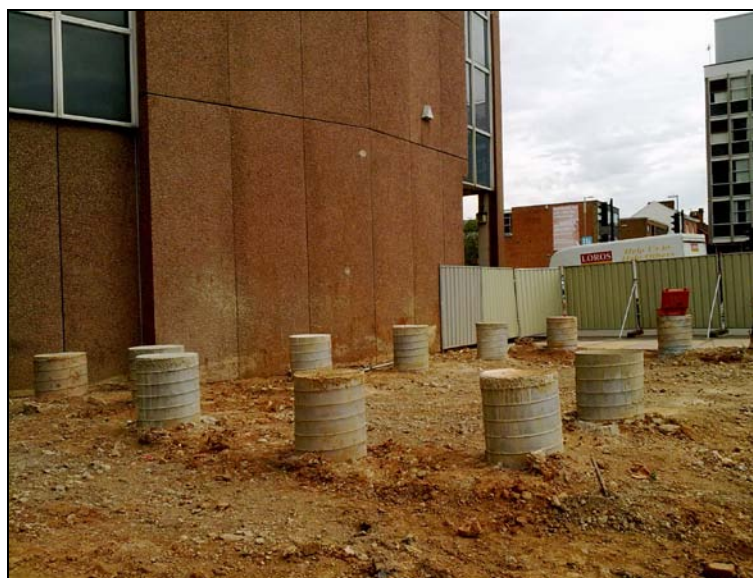
Figure 4: The completed piled foundation box showing pile caps
