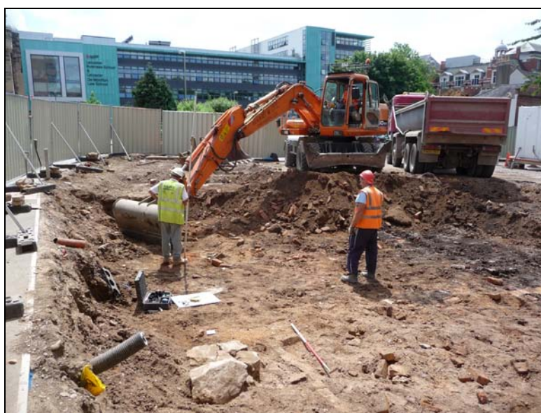
Figure 2: Machine clearance of modern overburden
