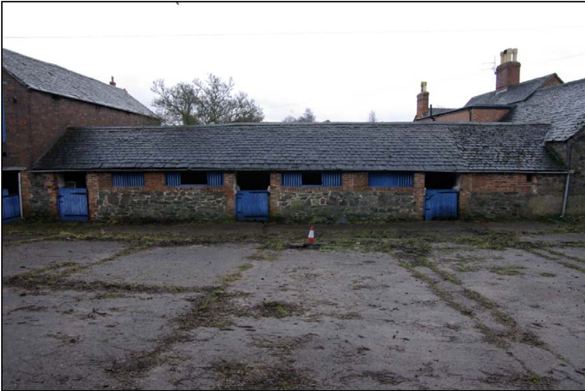
Figure 7 Building A1, principal elevation, looking south east (001-002).
