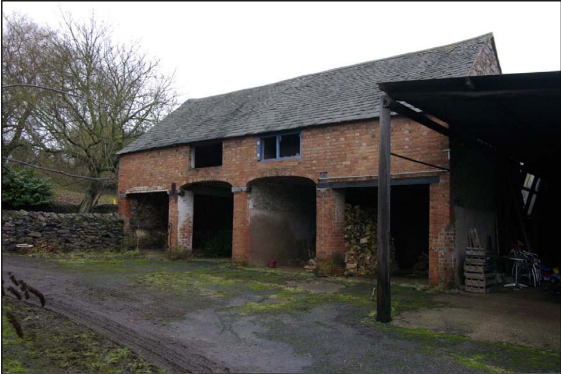
Figure 13 Building B, principal elevation, looking north-north west (091-092).
