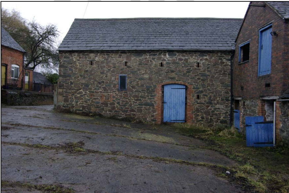
Figure 8 Building A3, principal elevation, looking north east (003-004).
