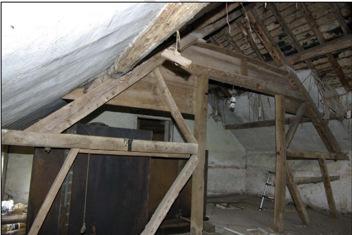
Figure 14 Interrupted tie beam truss, building B (116-117).
