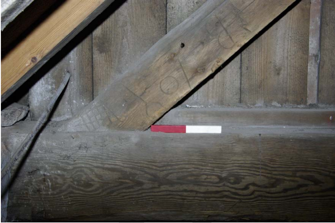
Figure 11 Rase or shipping marks on truss within A3 (059-060).
