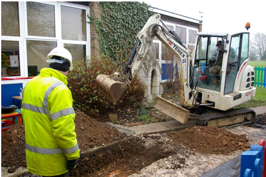
Plate 4: Work in progress on Trench 02, looking north-east
