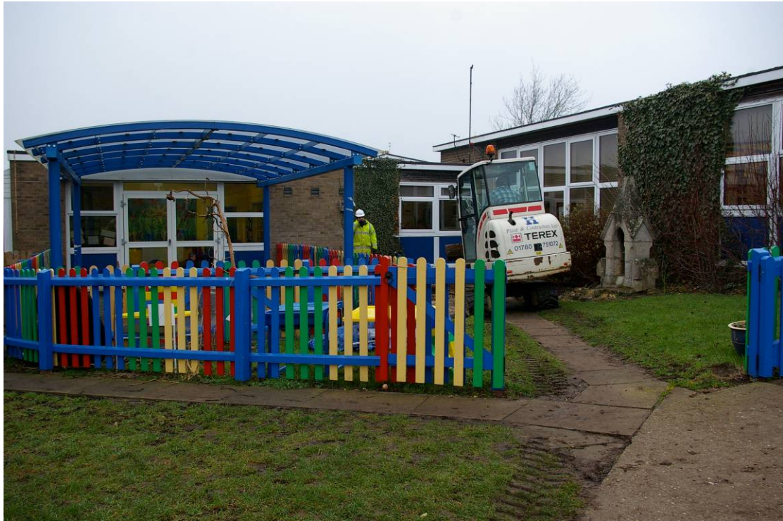
Plate 3: Location of Trench 02 at rear of school building, looking north-west
