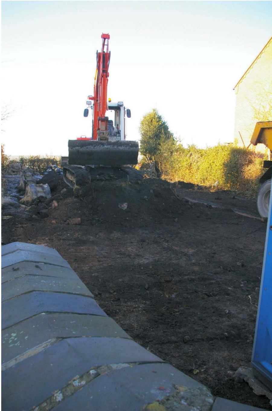
Figure 3 Proposed development area, work in progress (looking south-west).
