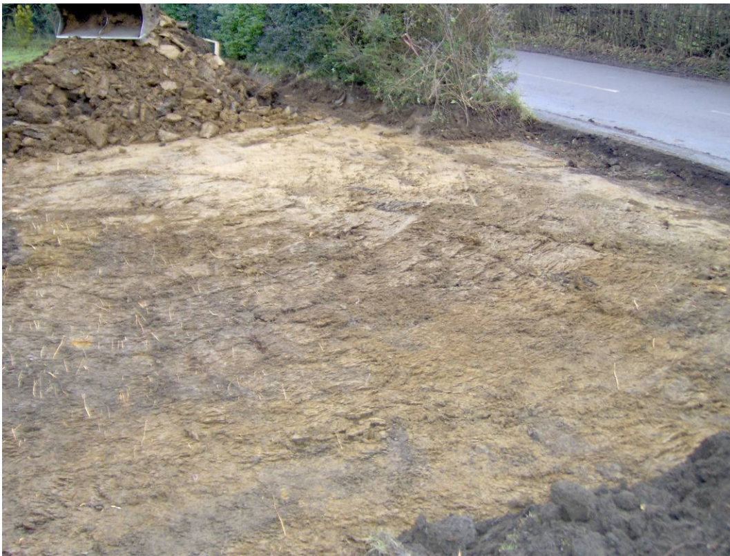
Plate 2: The street frontage stripped to natural clay, looking north-east
