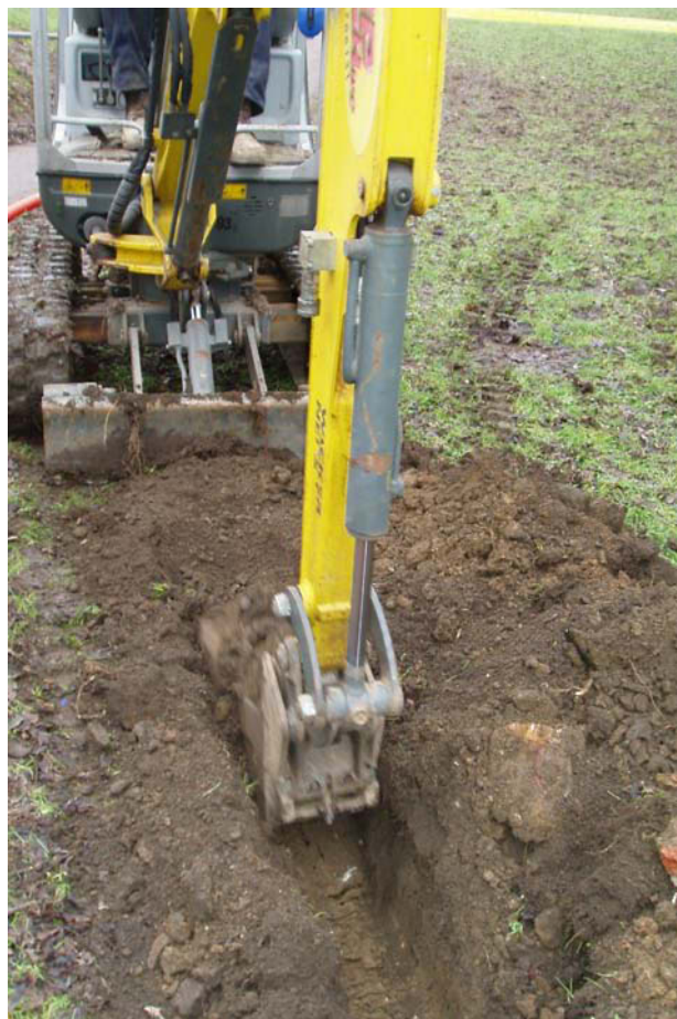
Figure 3 Cable trench under excavation
