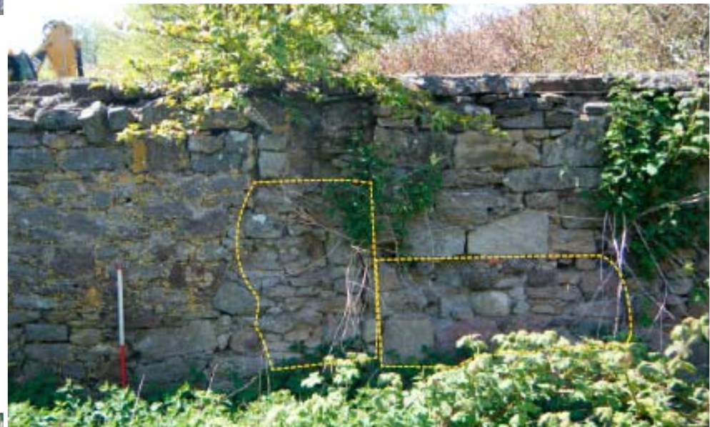
Illus 8 NE facing elevation showing F6 (left) and F5 (right)
