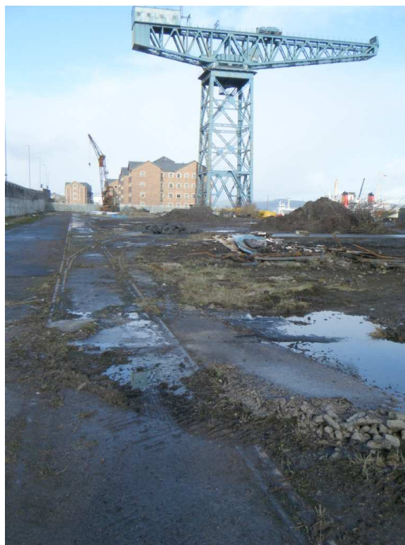
Illus 5: View of the listed cantilever crane
