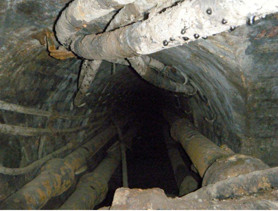
Illus 11: View of the service culvert and pipes
