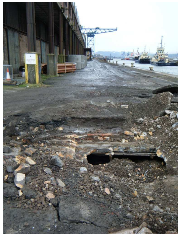
Illus: 10 Detail of the service culvert
