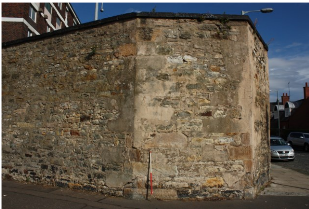
Illus 11: Boundary Wall , Portland Street
