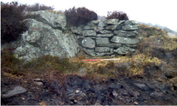
Grouse butt F20 at the N end of the area seen from S-W
