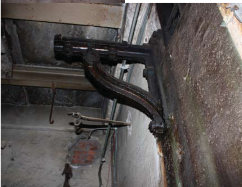
◀ Illus A10.12 Detail of the cast-iron support in Building I
