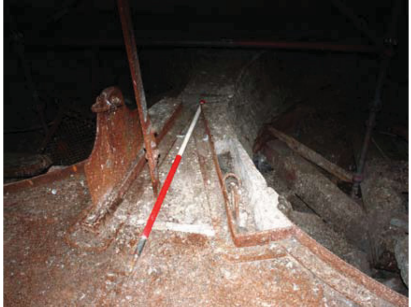
Illus A10.8 ▶ Detail of the lift plates of the mash tun furnace
