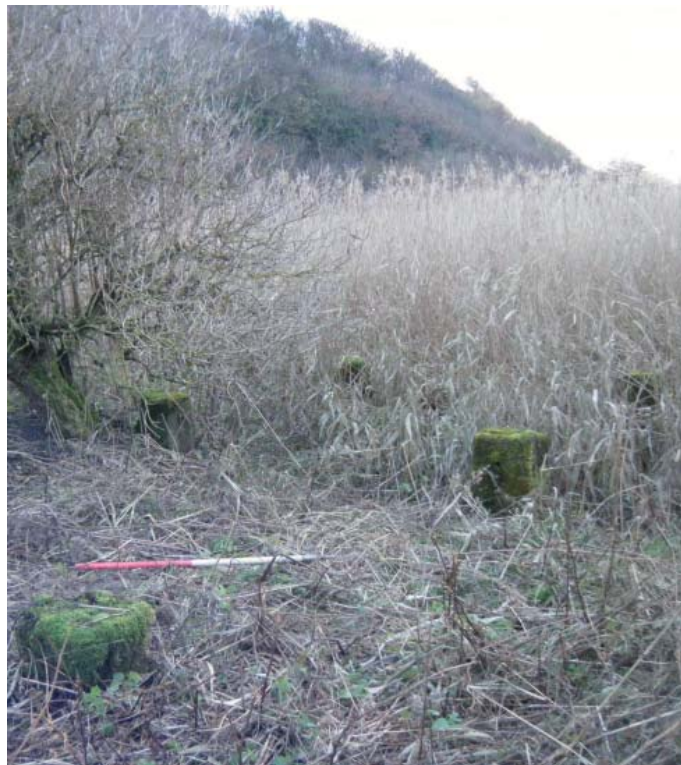
Illus 10 Concrete remains of pier
