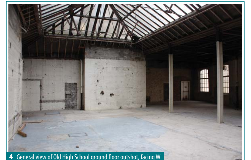
4 General view of Old High School ground floor outshot, facing W
