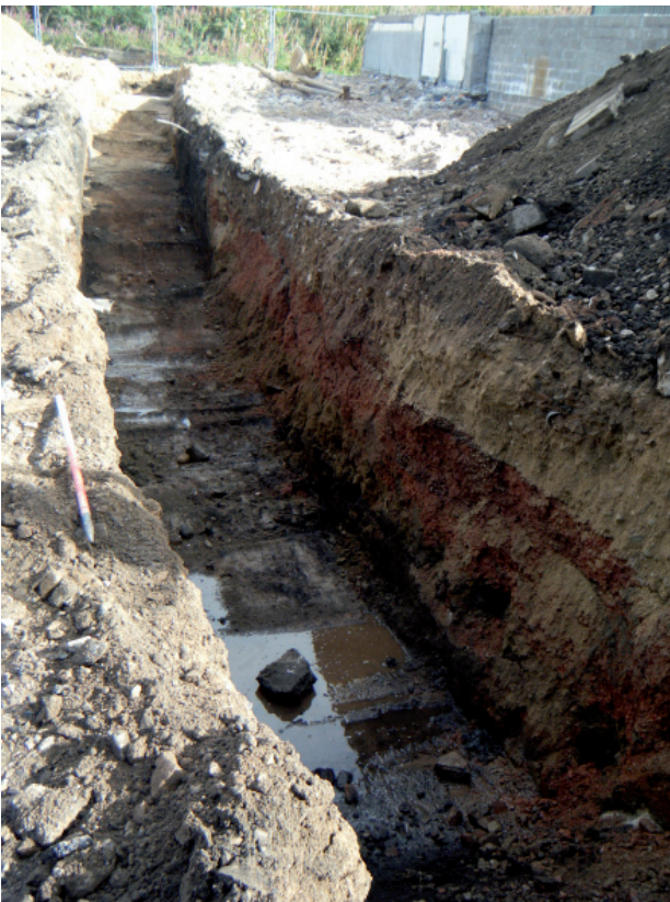
Illus 4 Deep demolition deposits in W-facing section at the south end of the Trench 3. From SW
