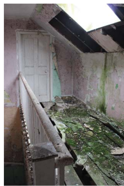
ILLUS 7B North range, first floor, hallway, general shot (044)
