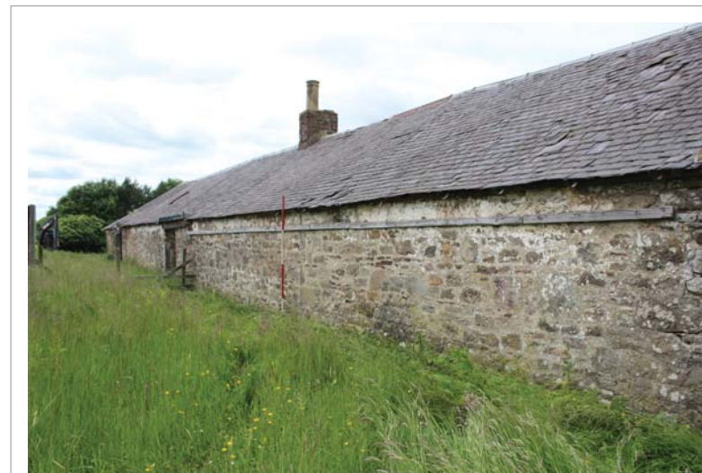
ILLUS 13B South range, south elevation, general shot of east end (049)
