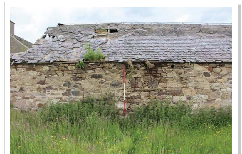
ILLUS 12C West range, west elevation, possible blocking (072)
