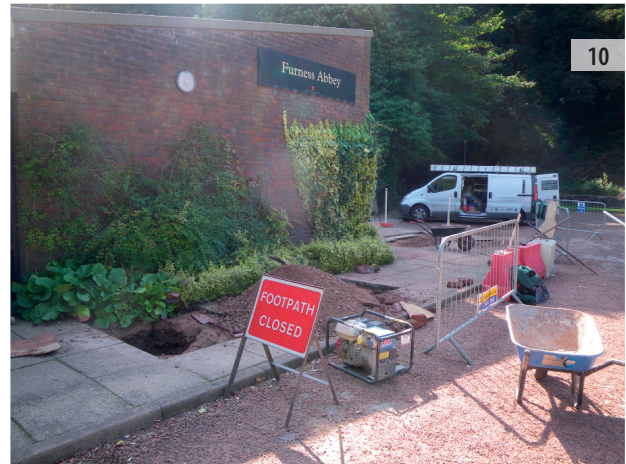
ILLUS 10 SW view of Trenches 5 and 6
