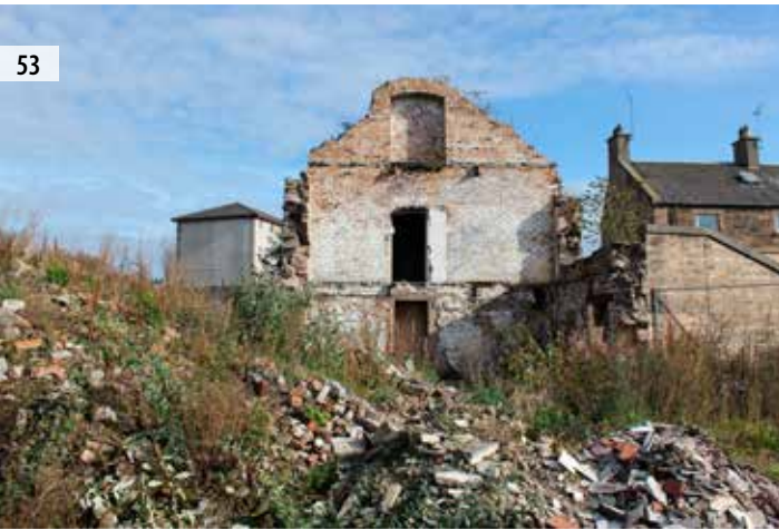
PHOTO 53 Gorgie Mill, general view of south-west external elevation
