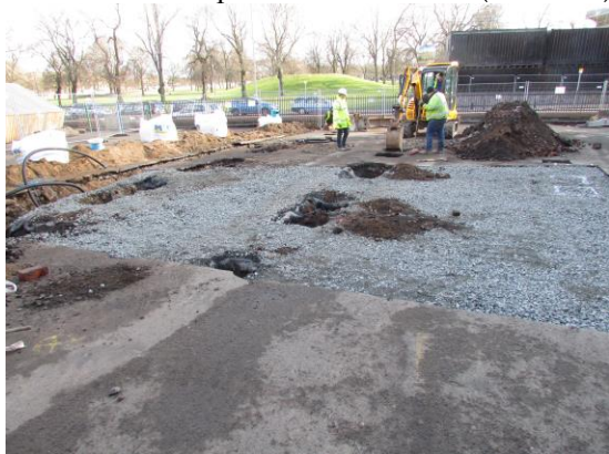
Illus 7 General view of the pad foundation excavations facing east
