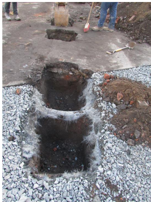
Illus 8 Detail of the pad foundation sections
