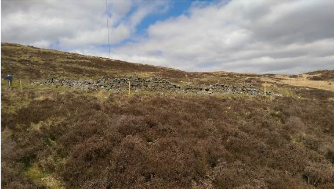
Figure 3: Southern upstanding element of wall, facing north.
