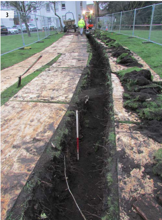
ILLUS 3 Eastern end of cable trench fully excavated
