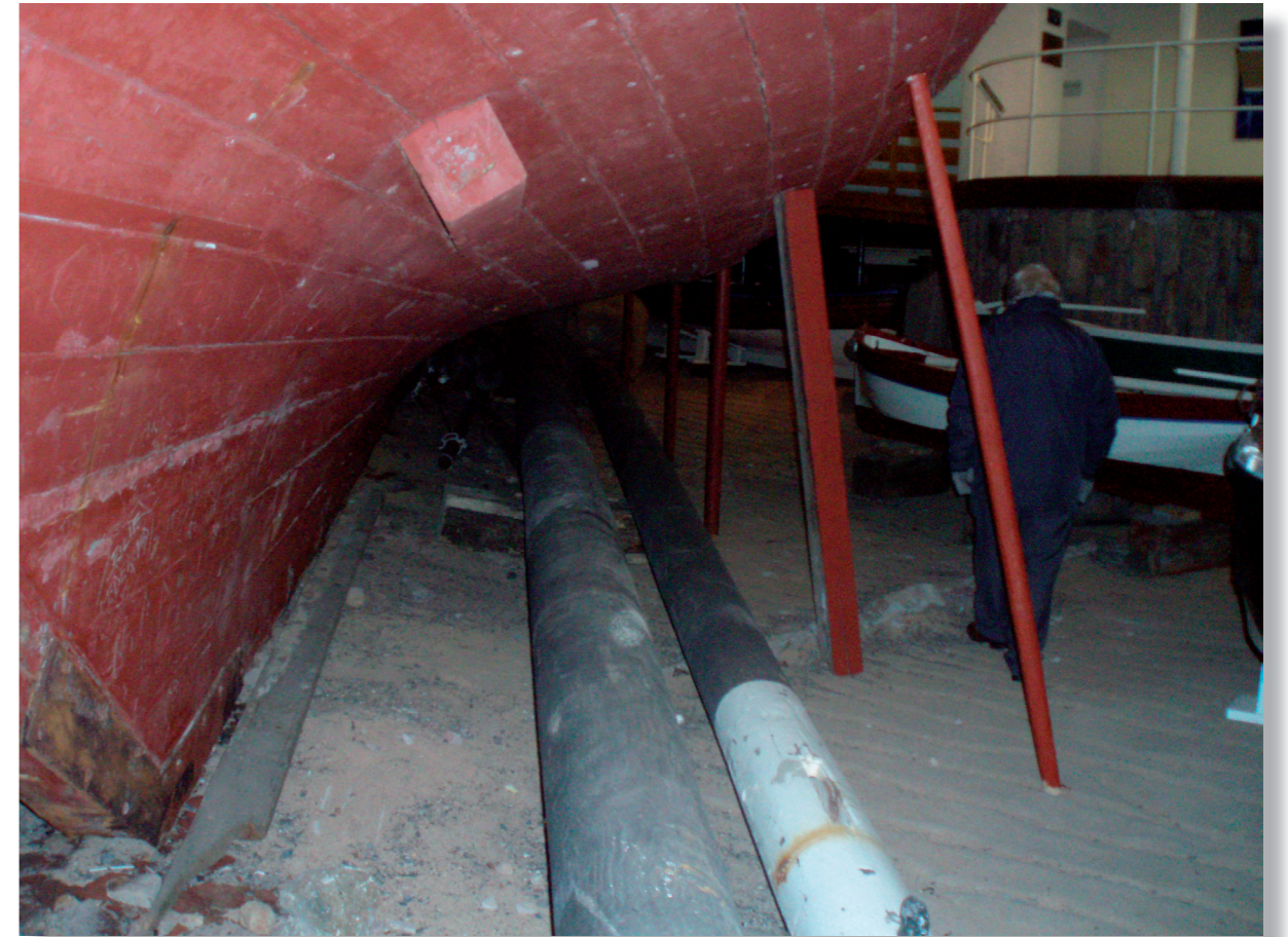
Illus 2c View along the starboard side of the vessel showing the current support technique for the hull
