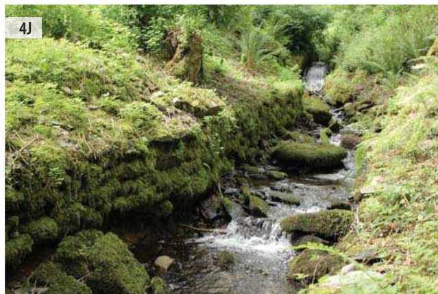
ILLUS 4 Site plan ILLUS 4A E facing view of sluice gate ILLUS 4B E facing view of newly exposed lade branch ILLUS 4C NW facing view of damage to northern side of weir ILLUS 4D SW facing view of damage to southern side of weir ILLUS 4E W facing view of rubble downstream from weir ILLUS 4F NW facing view of rubble in lade ILLUS 4G SW facing view of outflow lade from mill ILLUS 4H S facing view of previous consolidation works ILLUS 4I SW facing view of significant undercutting of lade walls ILLUS 4I SW view of undercutting of lade walls and related rubble
