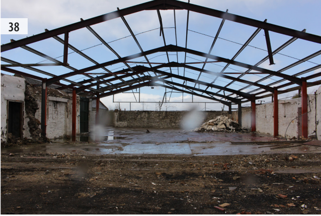
ILLUS 38 Interior of Shed
