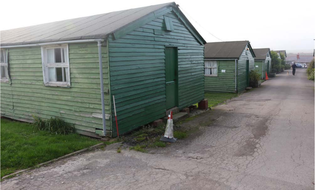
ILLUS 4 View of the site from the east ILLUS 5 General view of the southern row of structures
