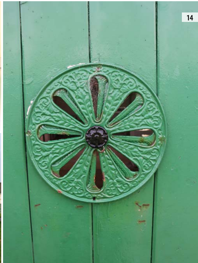
ILLUS 13 View of Block 6 ILLUS 14 Detail of cast-iron vent on the door of Block 6
