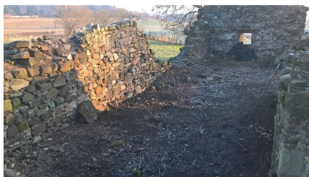
Illus 3 - Pre-excavation shot of the internal area of the church facing east
