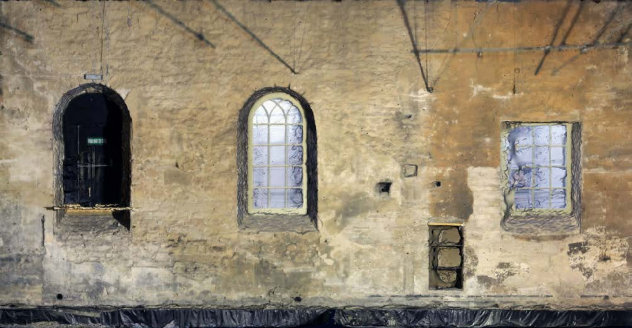
ILLUS 3 Quaker Meeting House – East elevation interior showing arched windows with blocked arch at south
