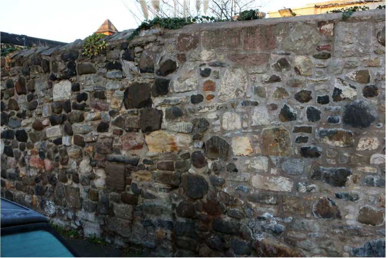
ILLUS 4 Start of rebuilding event of the southern wall. NW facing
