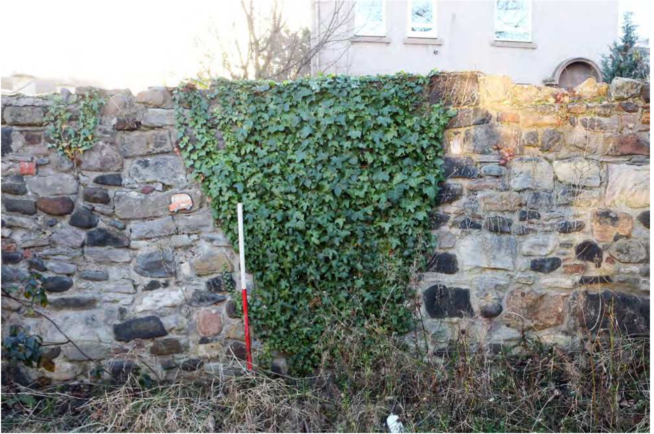
ILLUS 8 S facing shot of rebuilt wall section
