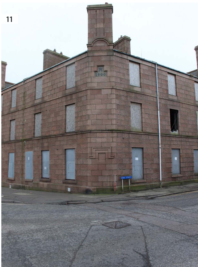
ILLUS 11 Detail of the original drip mould decoration and one of the later phase windows
