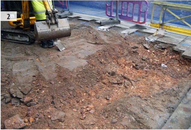
ILLUS 2 Working shot showing sand levelling layer beneath slabs
