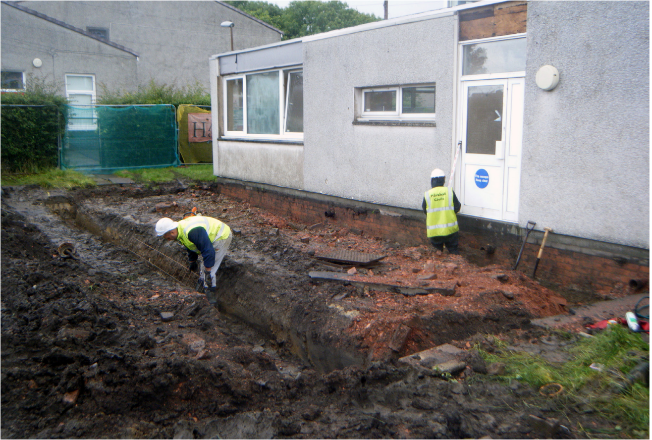
ILLUS 2 NW facing general shot of foundation trench area
