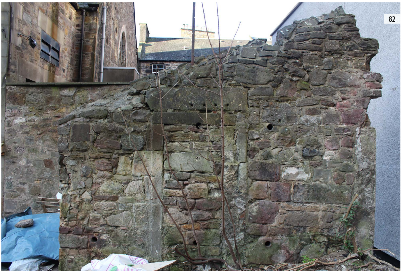
ILLUS 81 North facing elevation of Cowgatehead Church ILLUS 82 Shot of remnant wall segment relating to Pollock's Close
