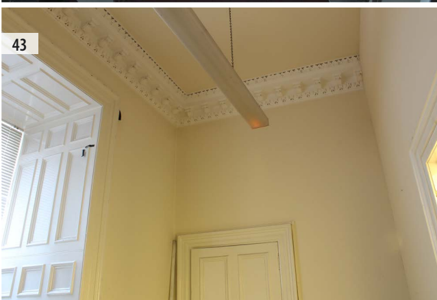
ILLUS 38 Elaborate corning (I1, 3) ILLUS 39 Domed roof and balconies within atrium (I1,10) ILLUS 40 Rounded room wall shared with atrium (I1,12) ILLUS 41 Victorian tile flooring of the atrium ILLUS 42 Victorian tile flooring from first floor atrium into hallways (I1,13) ILLUS 43 Corning with later dividing wall (I1, 1) ILLUS 44 Bay windows facing onto Victoria Street (I1,19)
