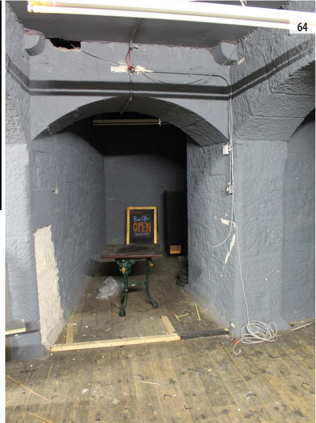
ILLUS 63 Bricked-up arch separating 4 India Buildings from 1-3 (I-2,1)
