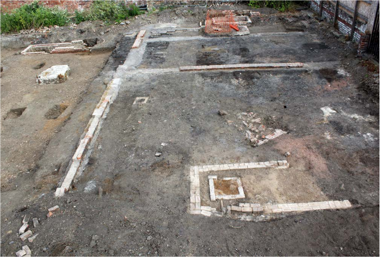
ILLUS 8 Basal brick courses on top of concrete wall foundations in east half of the North Area. Facing NNW
