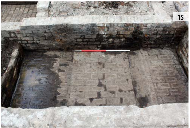
ILLUS 13 Block of concrete spanning pits [211 and 212]. Facing WNW ILLUS 14 Block of concrete in north-east corner of pit [174]. Facing north-east ILLUS 15 Traces of three removed division walls in pit [171]. One single brick wall near the middle of the scale and two double brick walls at either end of the scale. Facing NNW
