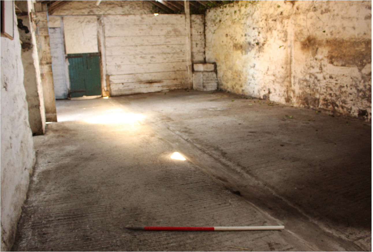
ILLUS 11 Internal view of Unit 2
