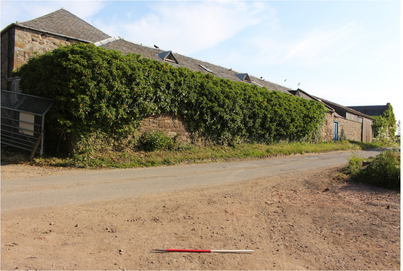
ILLUS 10 South facing elevation of Unit 2
