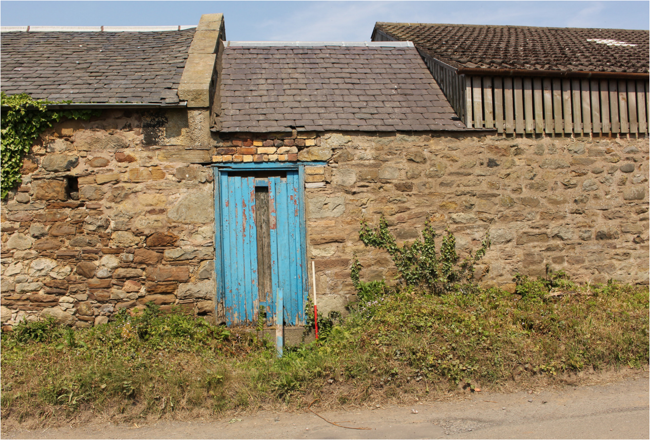
ILLUS 14 South facing elevation of the annex attached to Unit 3
