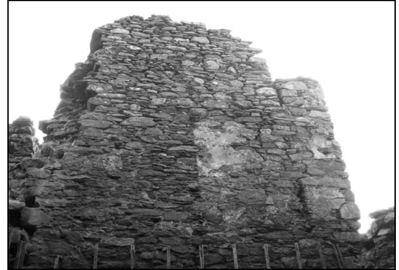
Plate 14 - Interior, NW block, mid-gable from NE
