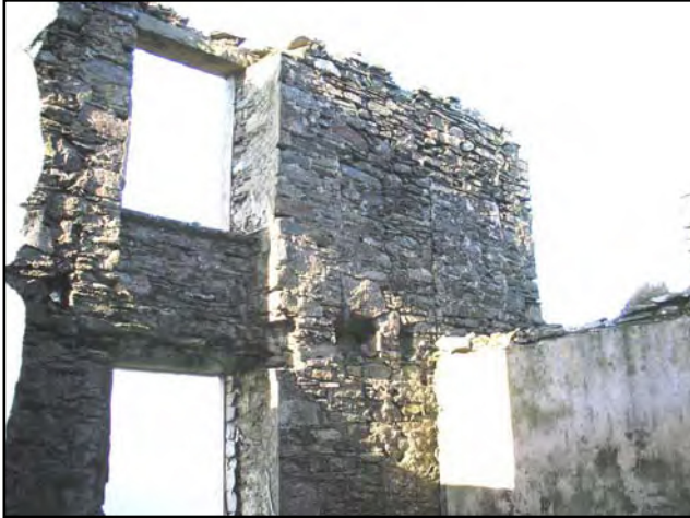
Plate 21 - Interior, SE block, SE wall, detail of joint between phase 2 and 3
