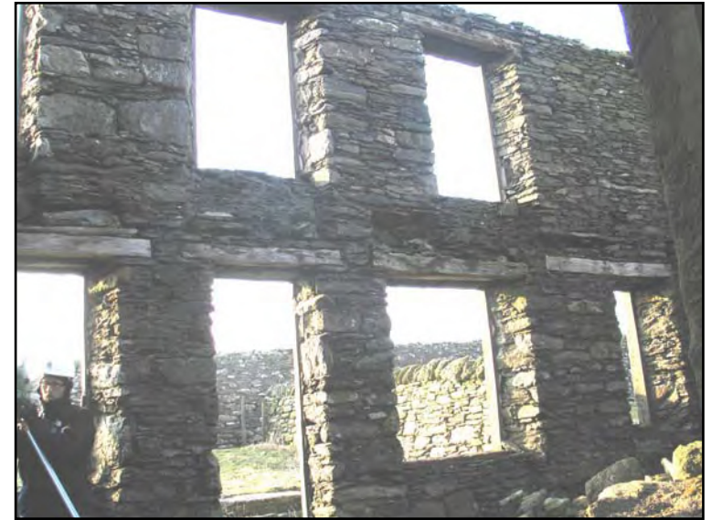
Plate 24 - Interior, SE block, SE wall of phase 3
