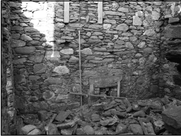
Plate 13 - Interior, NW Block, NE room
