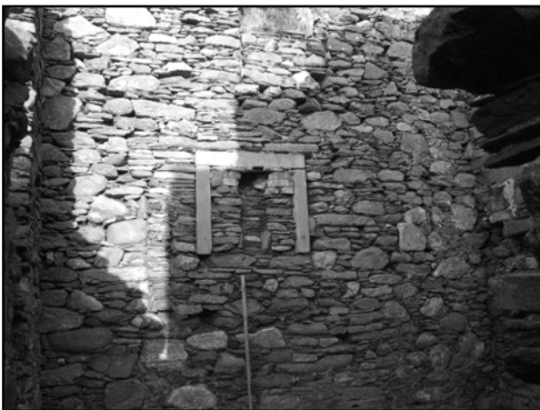
Plate 15 - Interior, NW block, NE room
