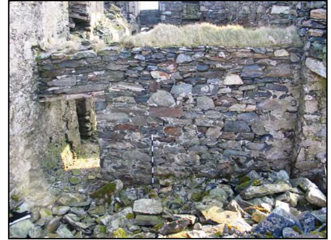
Plate 22 - Interior, SE block, partition wall in phase 2 block
