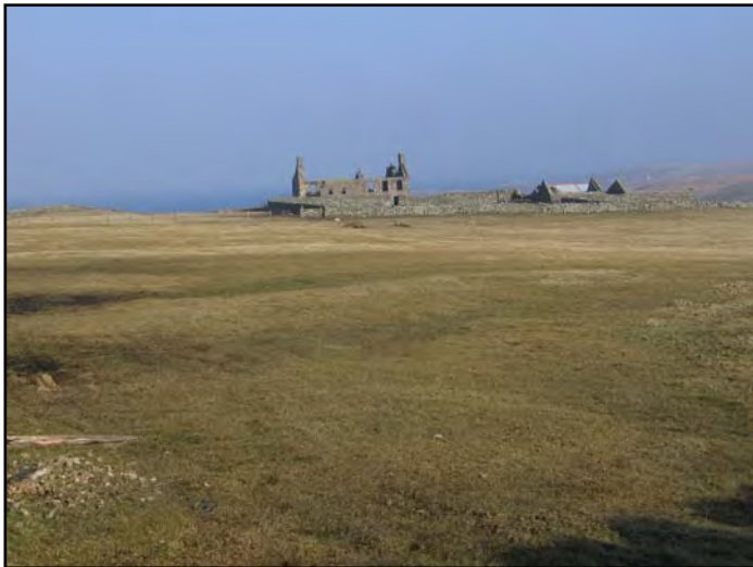
Plate 3 - view of the house, steading and the walled garden from the S
