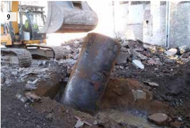
ILLUS 7 View of stone-lined culvert ILLUS 8 Detail of stone foundation with cut profile ILLUS 9 View of the fuel tank excavations ILLUS 10 Trench 1 facing east
