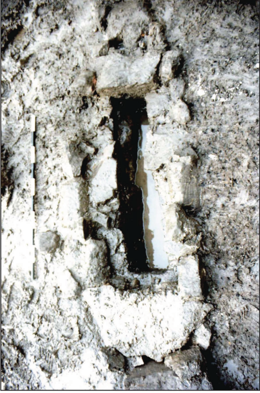
Plate 6: Plan of culvert with capstones removed looking SW
