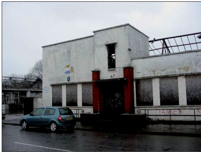
Plate 1: N facade, E entrance.
