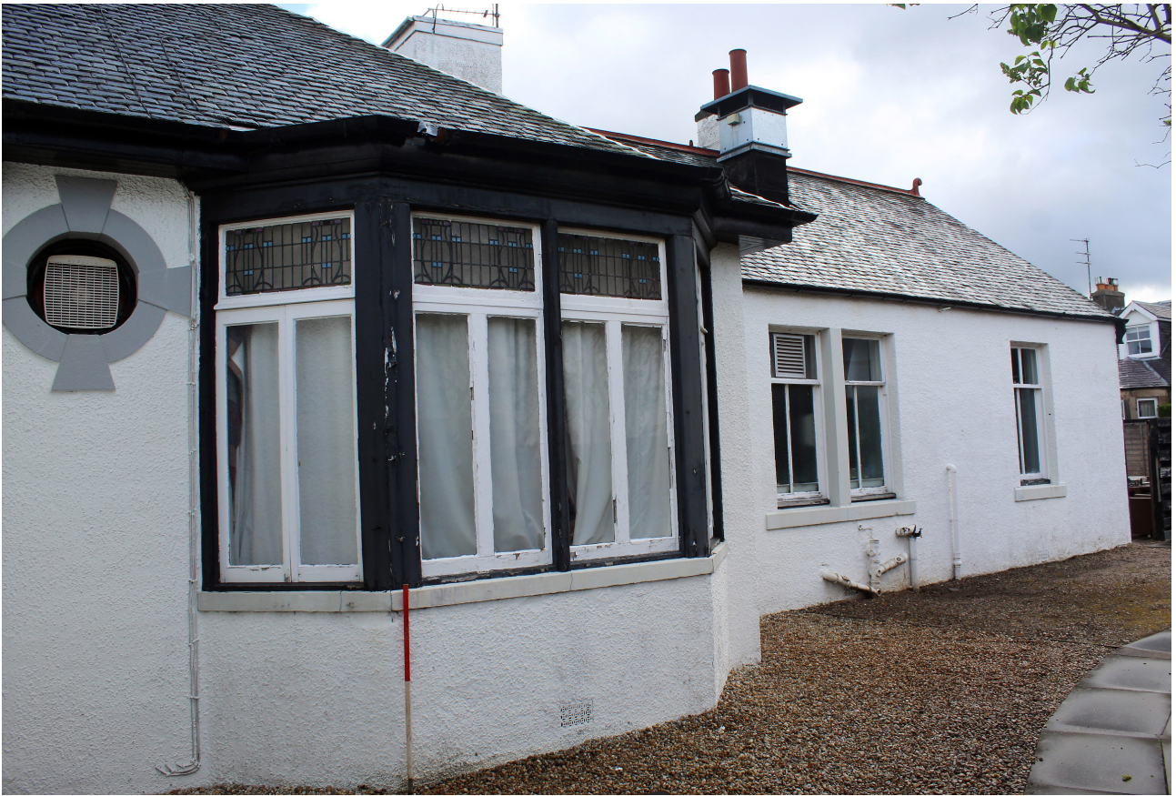
ILLUS 7 Detail of the art-deco window panes and ox-eye window on the south-west elevation
