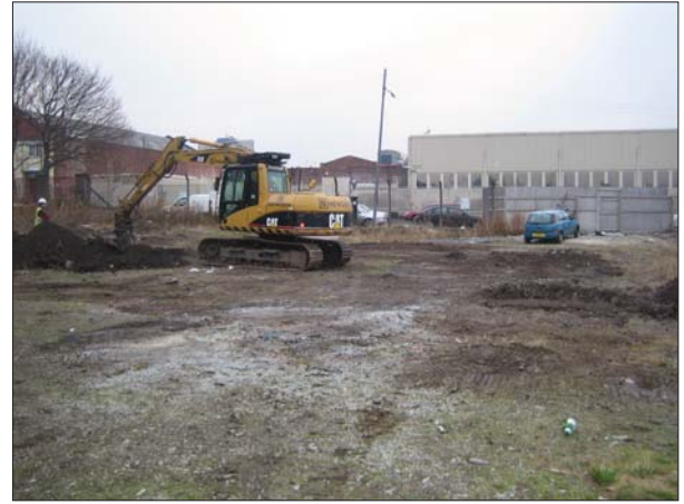
Plate 2 - Northern area of site, facing east
