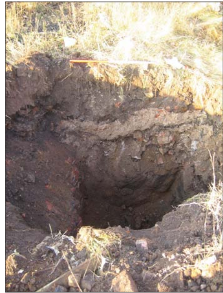
Plate 4 - Test Pit 1, with brick foundation 009.
