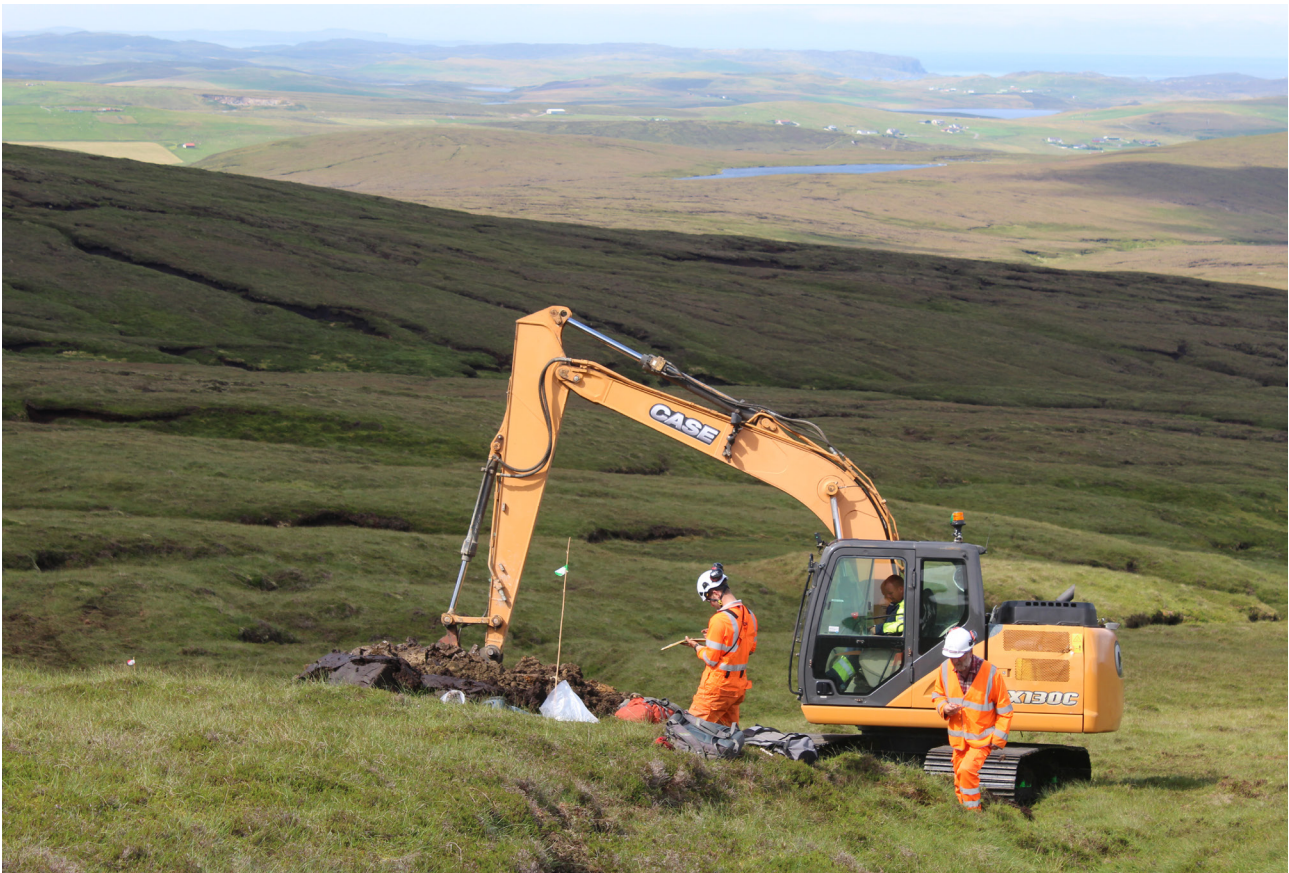
ILLUS 2 Machine excavation of trial pit
