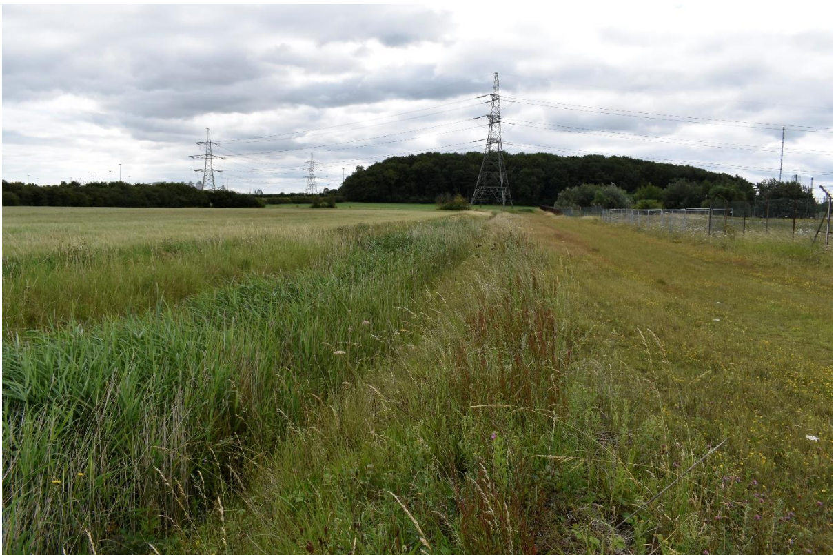
Figure 7. Ditch on eastern boundary of demolished Killingholme A power station.
