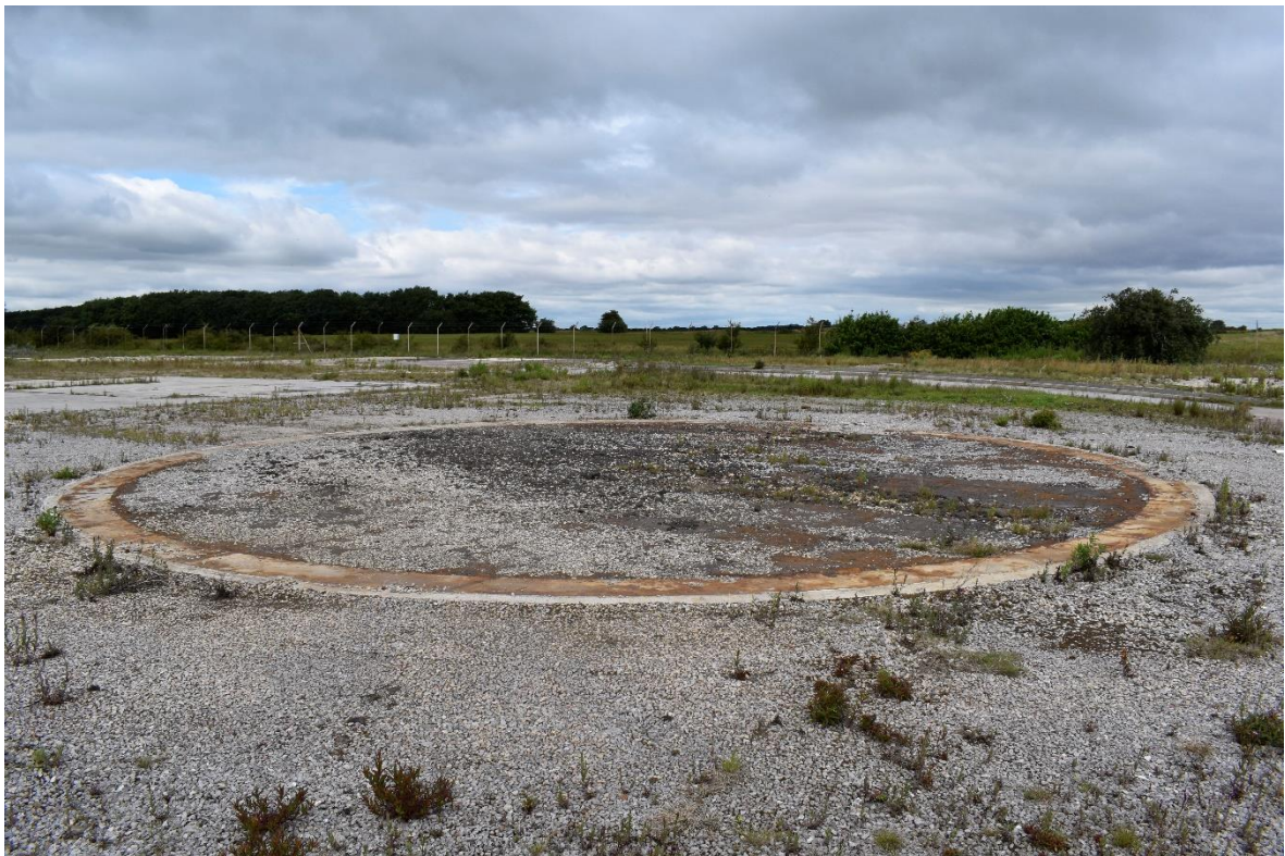
Figure 3. Remains of the demolished Killingholme A power station.
