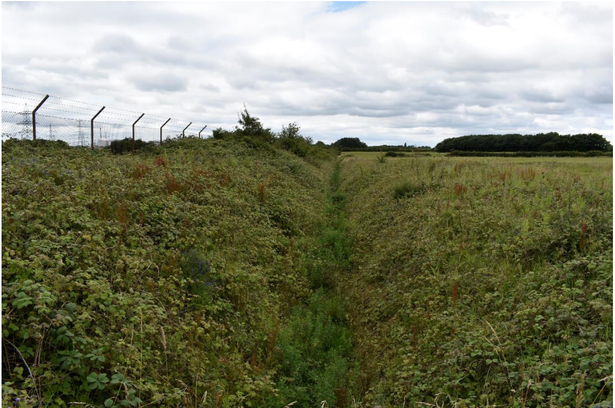
Figure 6. Ditch on northern boundary of demolished Killingholme A power station.
