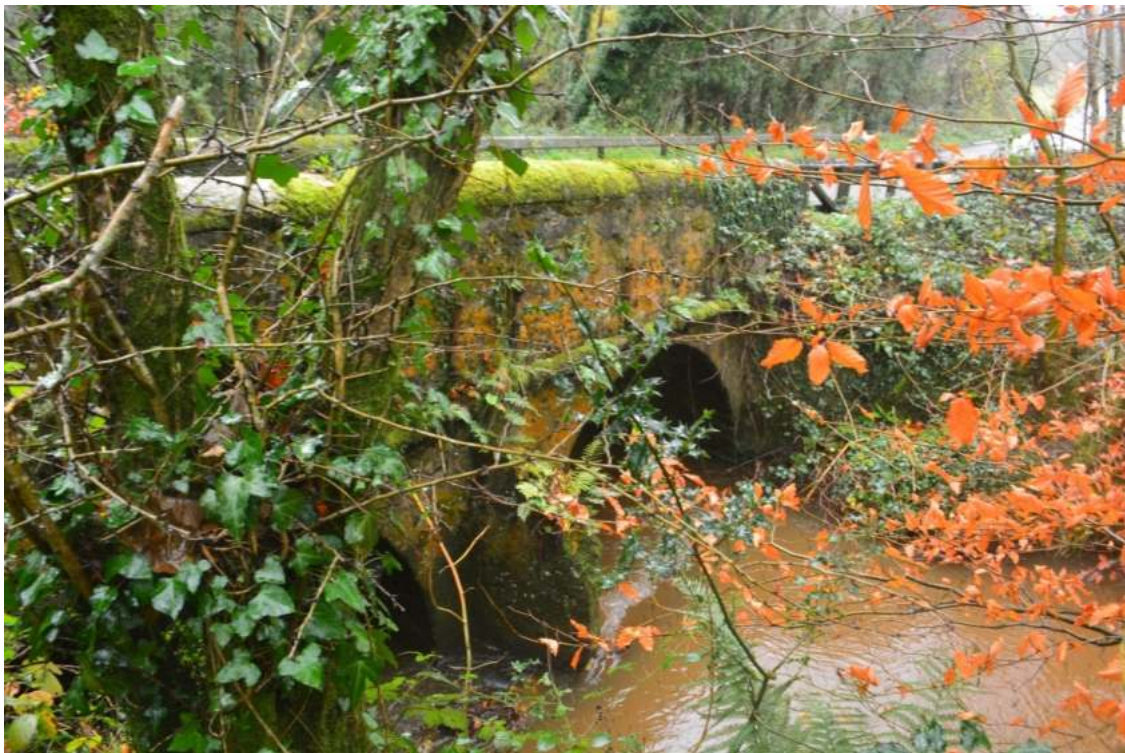
Plate 16: Trerice Bridge (LB 1144082)
