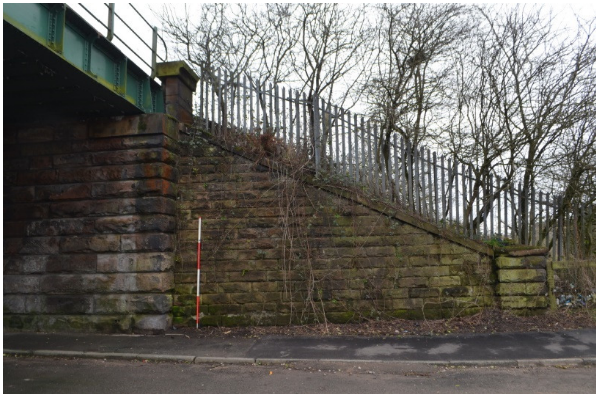
Illus 25. Underbridge 55, detail of north-western retaining wall.
