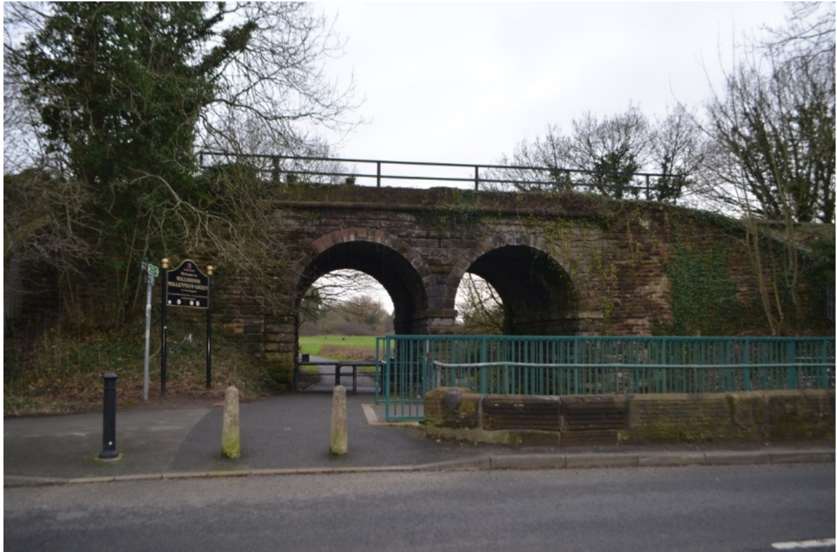
Illus 28. Underbridge 56, north facing elevation. Mill Bridge is in the foreground.
