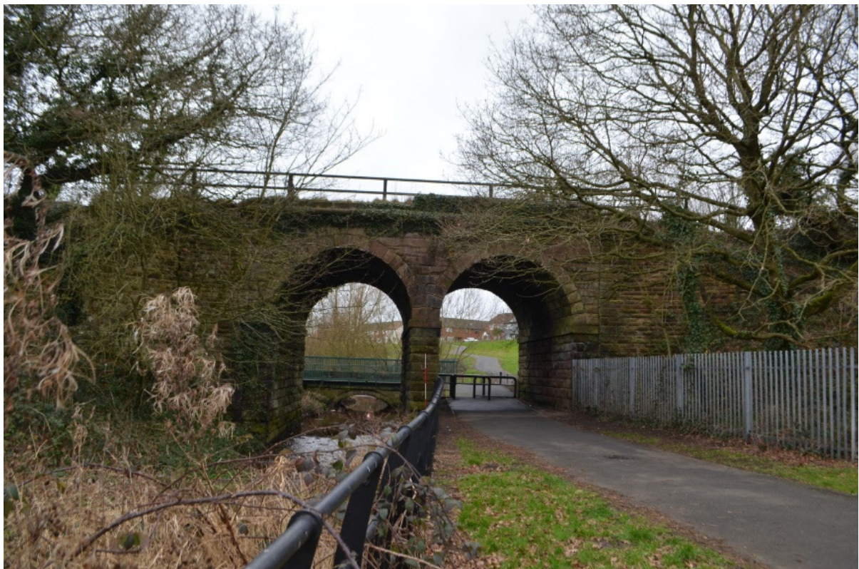
Illus 29. Underbridge 56, north facing elevation.
