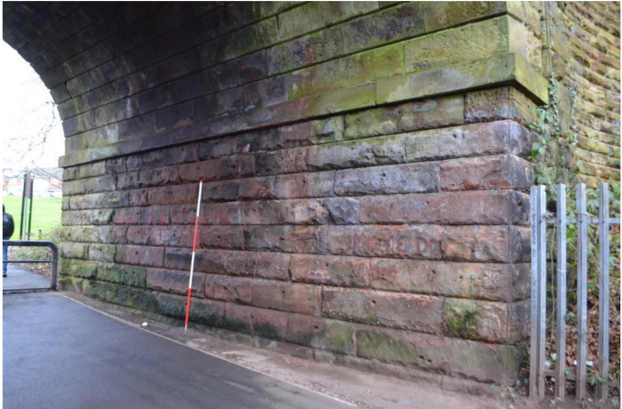
Illus 30. Underbridge 56, detail of eastern pier.
