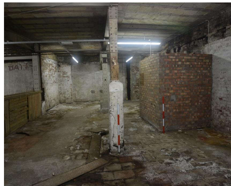
Illus. 6. South-western area of Room BM. 1, looking south
