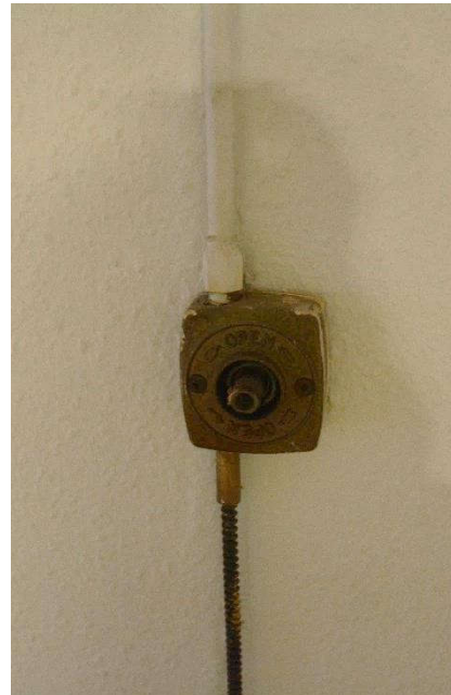
Illus. 59. Light switch attached to pillar in Room T. 3, looking west
