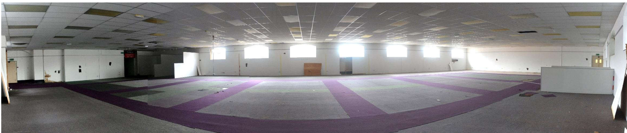
Illus. 78. Panorama of Room FIF. 3 from its southern side, looking west to east
