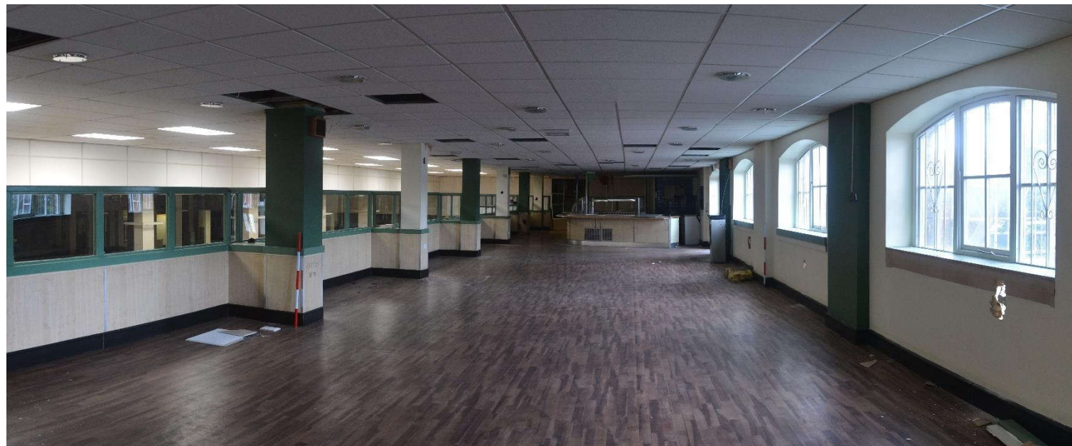
Illus. 45. Room FSTM. 3 from its eastern side, looking west
