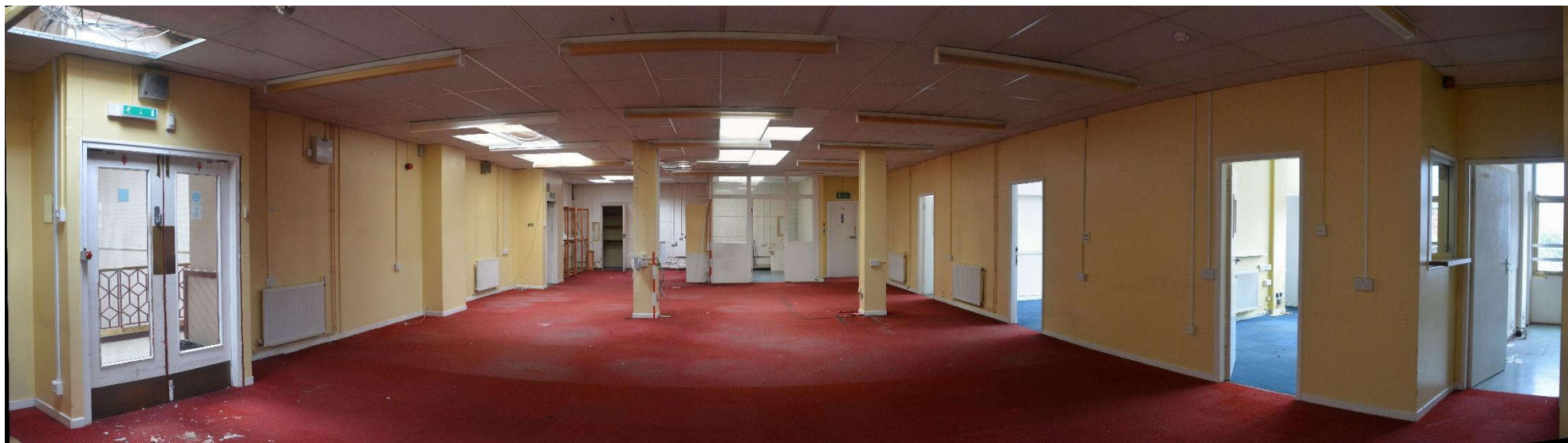
Illus. 85. Panorama of Room SI. 1 from its eastern side, looking south-west to north-west
