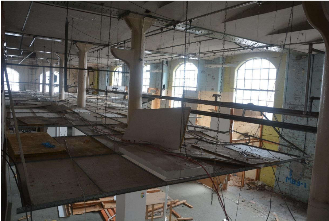
Illus. 55 (left). View of suspended ceiling in Room T. 1 from Room TM.2, looking east-south-east
