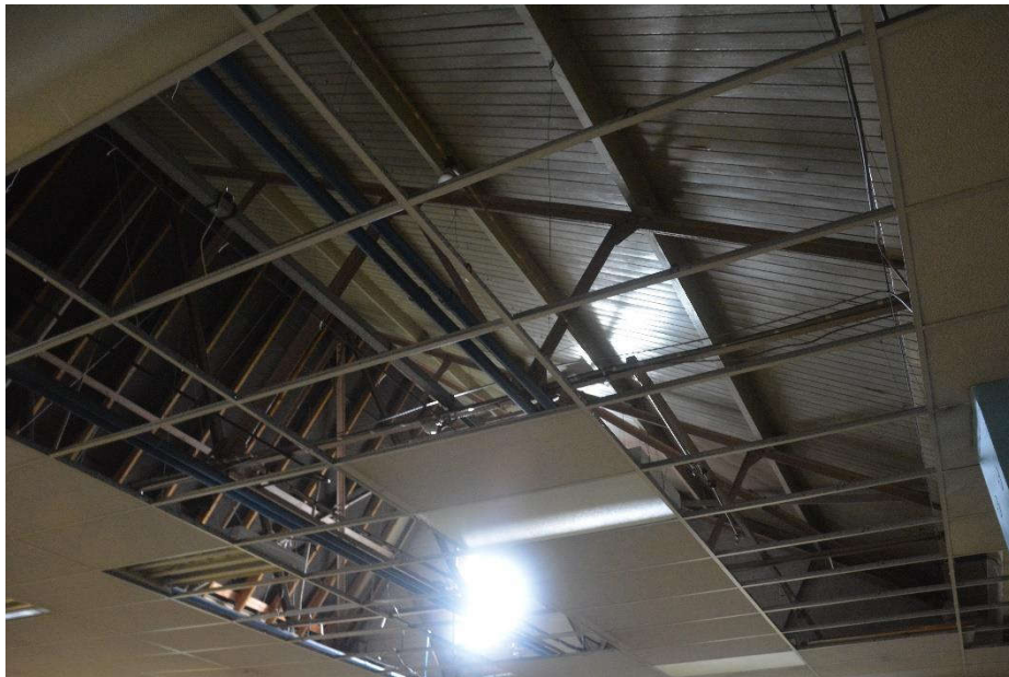
Illus. 58. Exposed roof of Room T. 3, looking north-east
