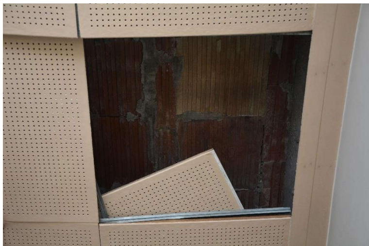
Illus. 92. Exposed earlier ceiling in Room SI. 6, looking south
