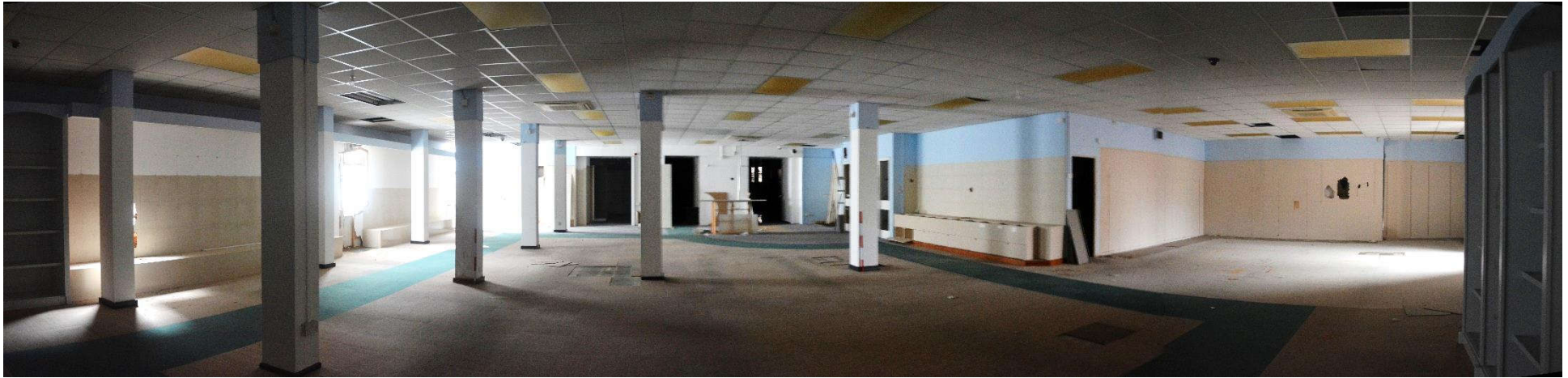
Illus. 50. Panorama of Room S. 3, looking north-east to south
