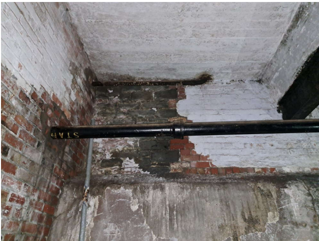
Plate 204a: West side of northern elevation in Basement room BM.2. Shows pennant wall with ash lime mortar, probably part of the 1811 factory. No scale
