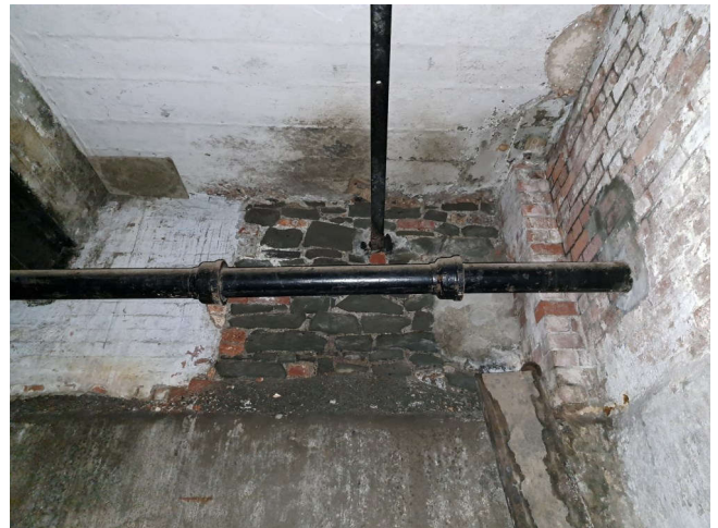
Plate 204b: East side of northern elevation in Basement room BM.2. Shows pennant wall with ash lime mortar, probably part of the 1811 factory. No scale
