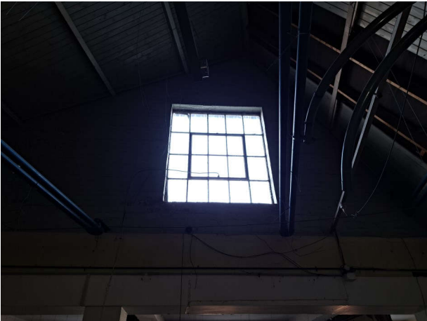
Plate 198: Phase 3 window in central gable of the western elevation of Building 3. No scale.
