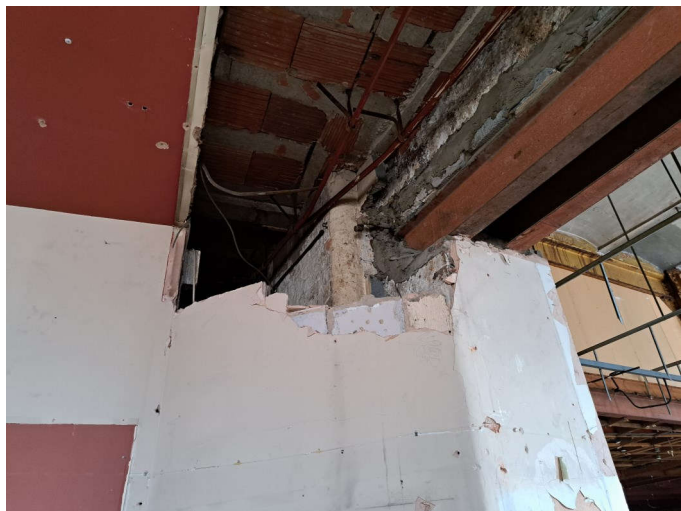
Plate 201: Area of exposed Phase 2 fabric visible in inserted opening into room FST.8. No scale
