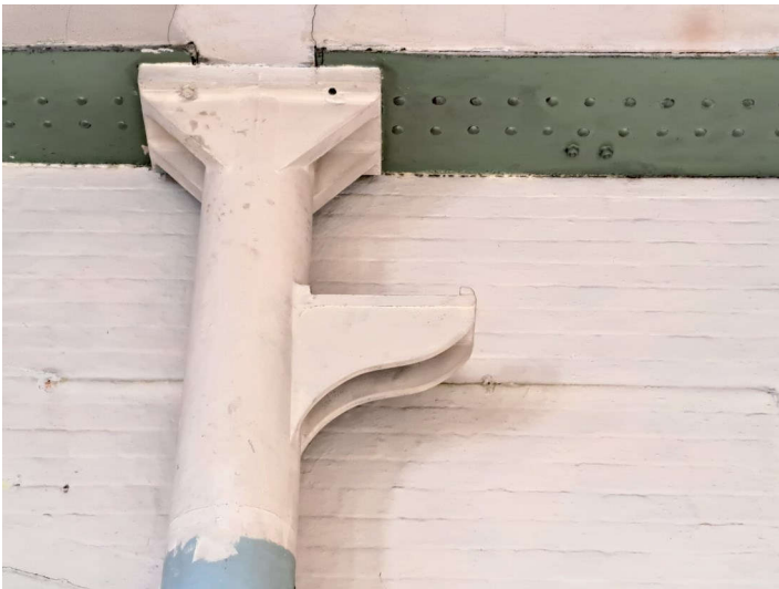
Plate 180: Detail of metal hook feature of central support columns in the western end of room T.1 (Building 1). No scale
